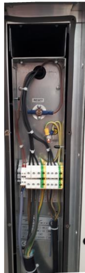
access to the heater connection terminal block - - after removing the front panel on the operating side of the unit
