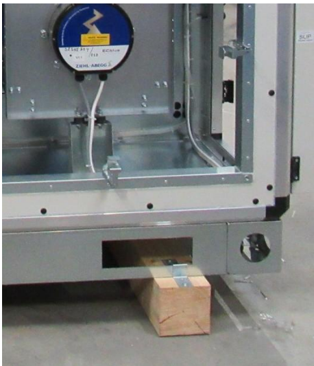
detail of the transport beam expedition blocks of DUOVENT® MODULAR DV/RV units
