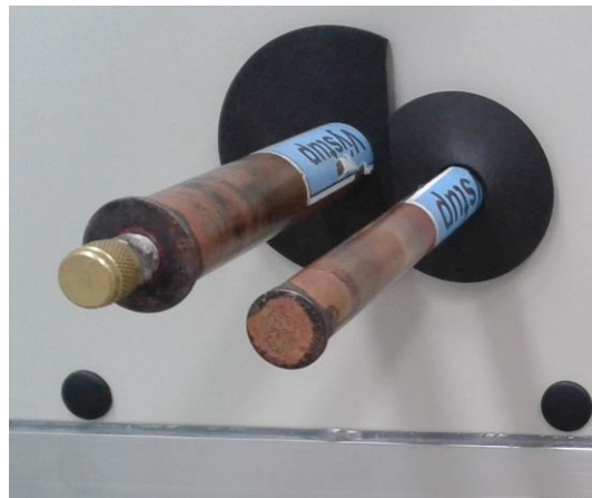
example of the design of the connection sockets of one direct evaporator circuit
